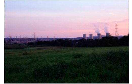
32. Three Mile Island, Pennsylvania, 30.8.1994
